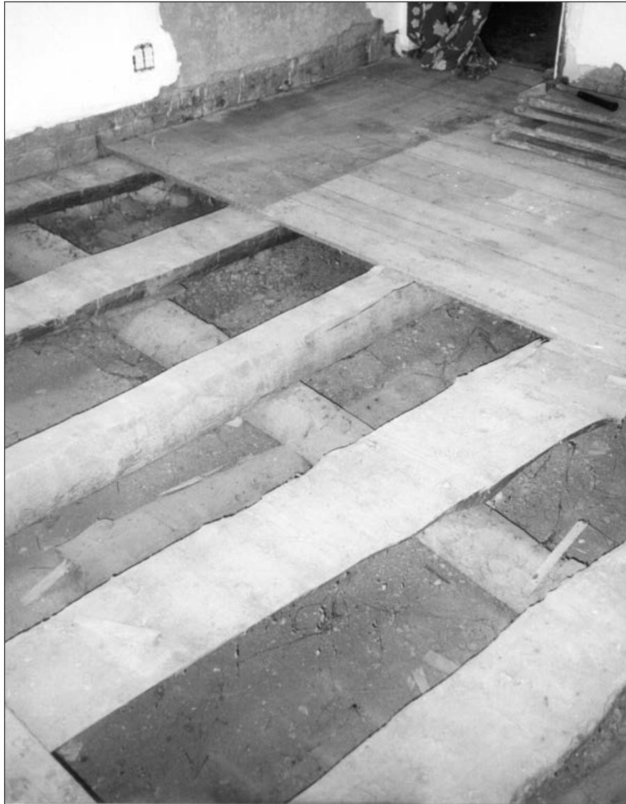
Figure 11. Photo of the central support beam floor in room block #2. The doorway leading to room block #4 is at the upper right.
