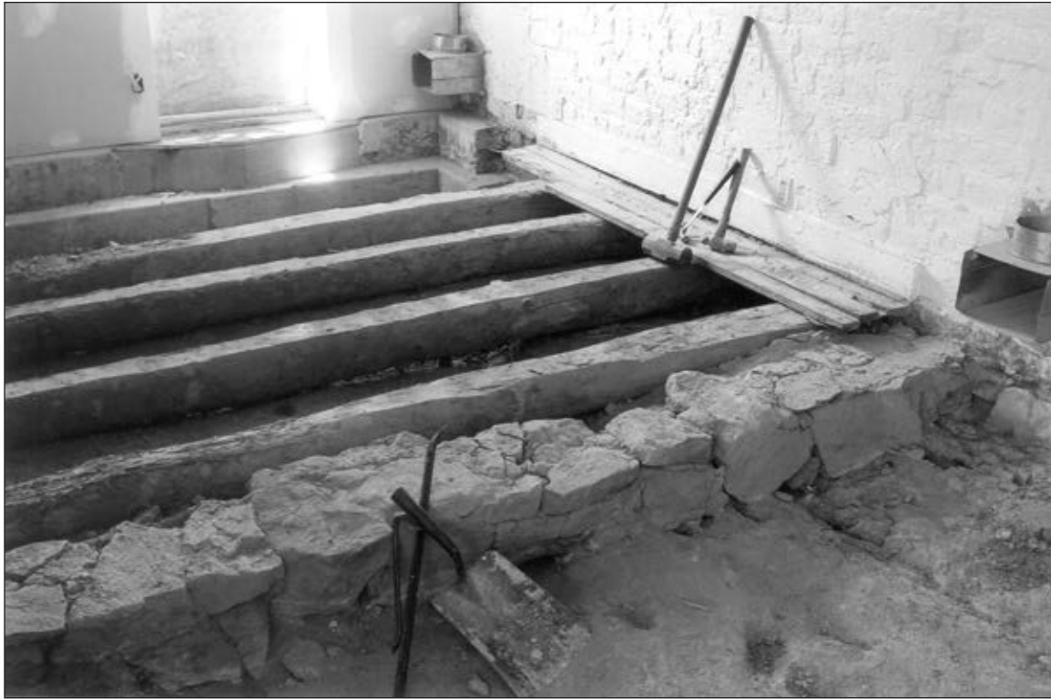
Figure 5. View from room block #4, of the log and plank floor being removed from room block #3. In the foreground is the interior dividing wall foundation, to the right is the central wall of the house. Upper left is the gable end wall that has been stabilized with a new concrete foundation.
